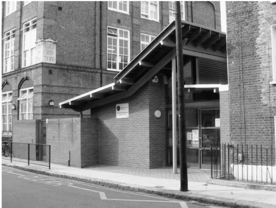
Image 9: Entrance from William Street
